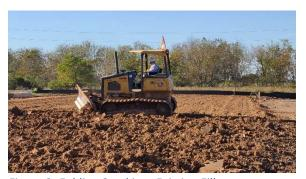
Figure 3- Folding Sand into Existing Fill
