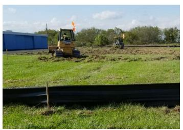
Figure 2 - Stripping topsoil for grading
