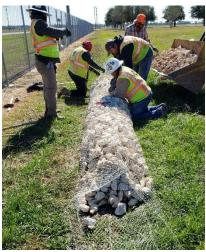
Figure 1- Installation of Filter Dam
