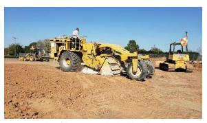
Figure 4 - Select fill mixing on the building foundation
